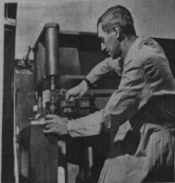
Foreman adjusts one of three jacks which will help maintain alignment of steel girder sections of the accelerator.
